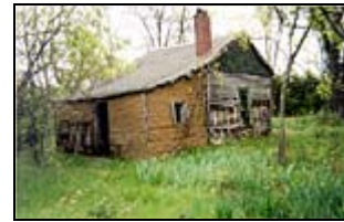
Second cabin, addition. Note brick chimney.
