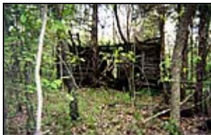
Small cabin (visible from the public road)--roof off; located on last property John Chilcoat lived on.
